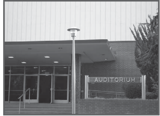
MJC's Auditorium project is one of the first on the schedule.
