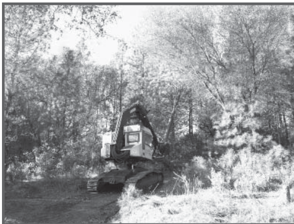
Clearing the way for the Columbia College Secondary (Emergency) Access Road.
