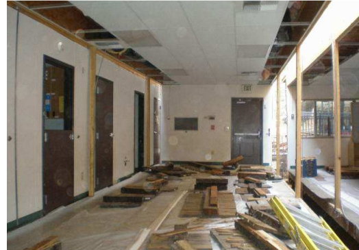
Pinyon Relocation Project construction
