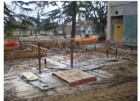
North Side Underground Plumbing
