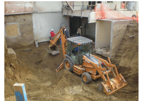
West Side Footing Excavation at Elevator
