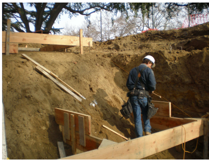
Installing Formwork for East Side Stairs
