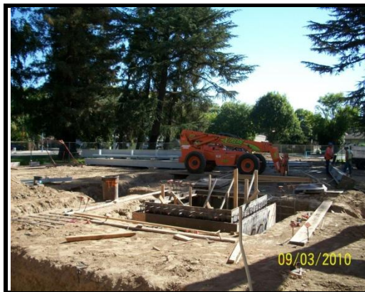
FORMING FOR ELEVATOR PIT CONCRETE
