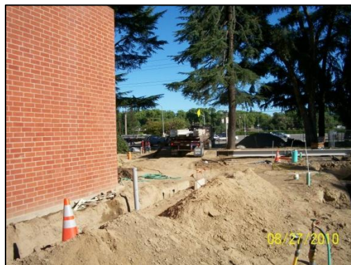
PLACEMENT OF ELECTRICAL CONDUIT AND GAS LINE
