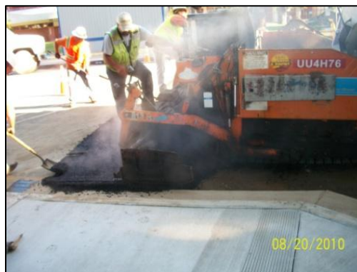
INSTALLATION OF ASPHALT CONCRETE IN PROGRESS
