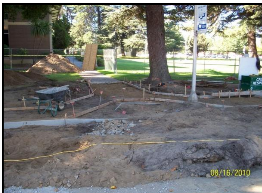
SIDE WALK FORM WORK IN PROGRESS
