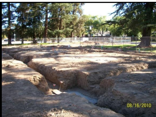
INSTALLATION OF COLUMN FOOTING CONCRETE
