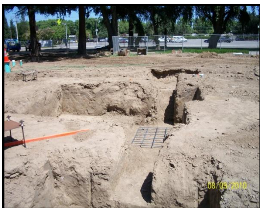
EXCAVATION FOR FOOTINGS
