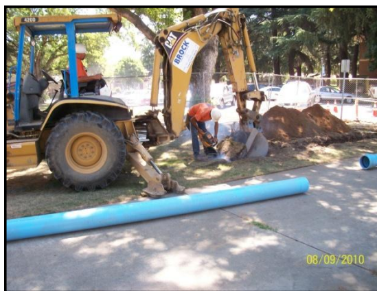
INSTALLATION OF WATER LINE PIPE
