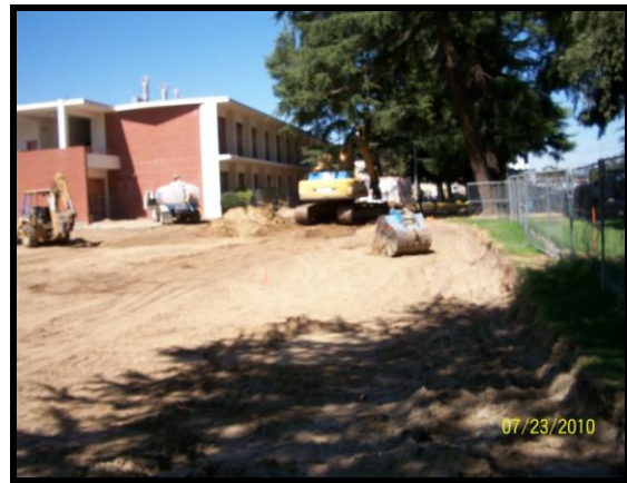
WORKING ON TRENCHING FOR FIRE SERVICE WATER LINE
