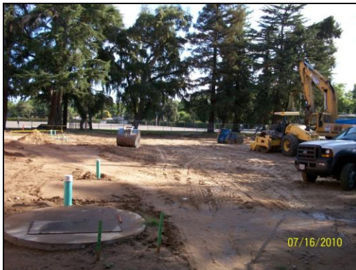
COMPACTION OF BUILDING PAD IN PROGRESS
