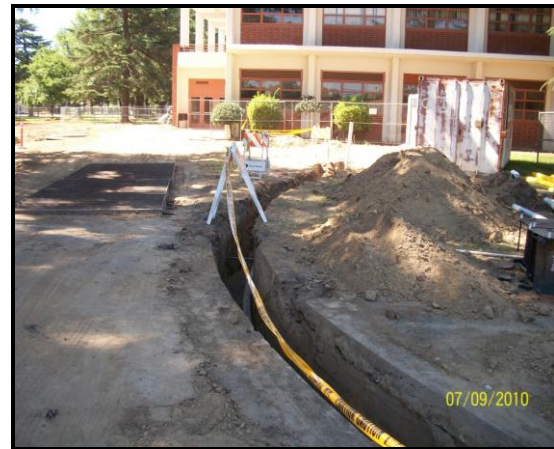
TRENCHING FOR ELECTRICITY
