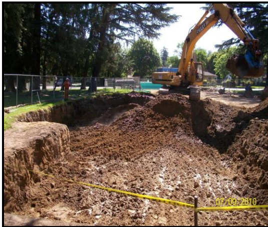
EXCAVATION FOR BUILDING PAD
