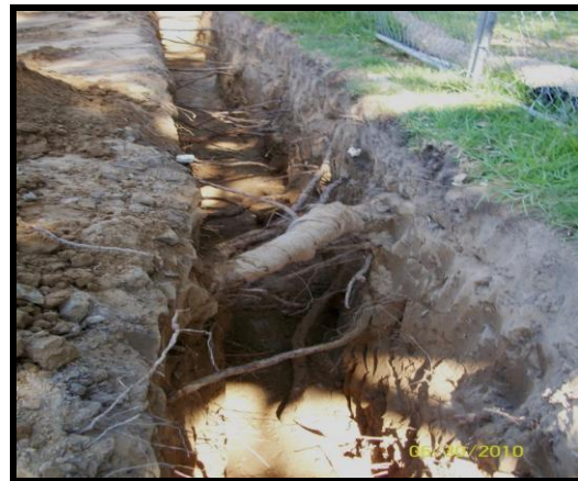
Excavation for utilities within tree drip lines by hand.
