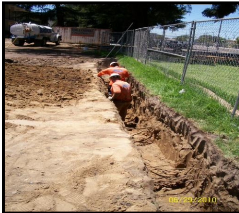
Excavation for utilities within tree drip lines by hand.
