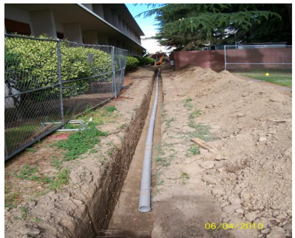
Storm water piping installation
