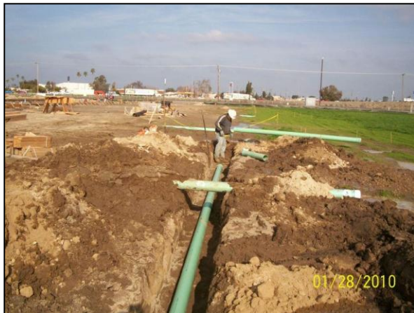
Installing Sanitary Sewer Pipe
