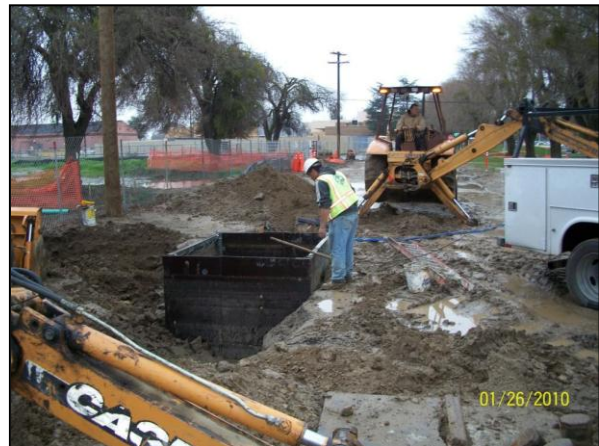
Installing Sanitary Sewer Manhole
