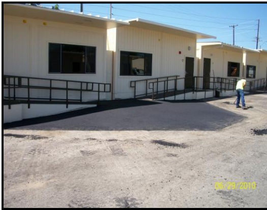
PORTABLE ACCESS RAMPS ARE BEING INSTALLED.
