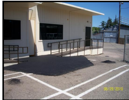
Portable access ramps are being installed.
