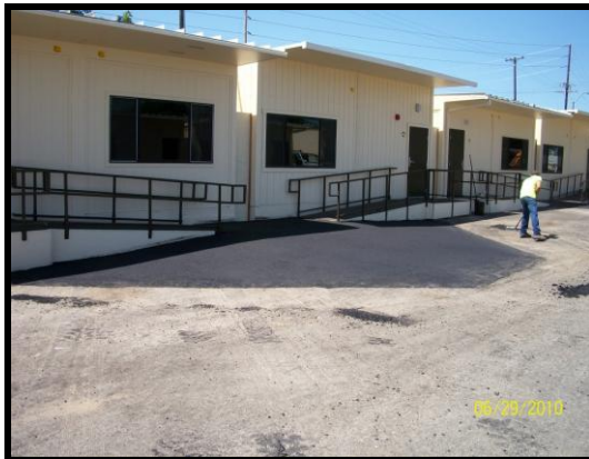
Portable access ramps are being installed.
