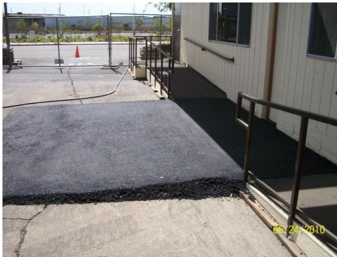
Access ramp installation in progress.
