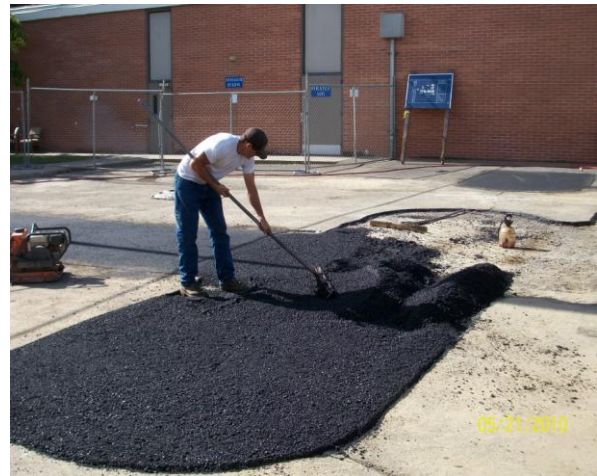
Final patch to asphalt
