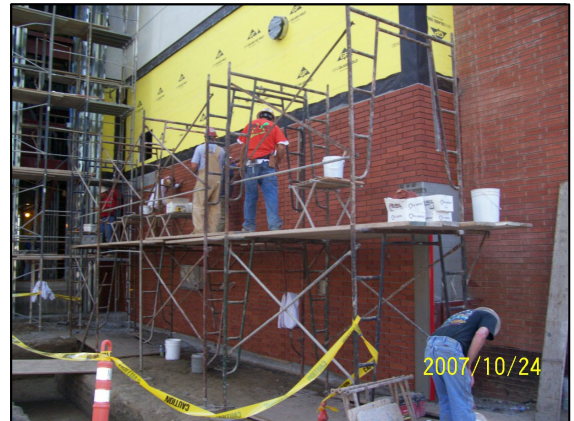
Installing Thin Brick at the South Side Addition
