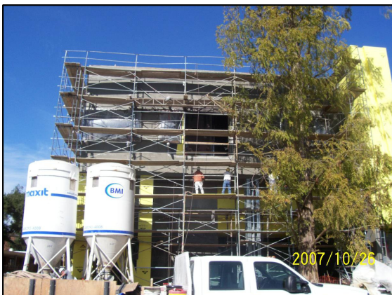
Plastering Exterior Walls at the South Side Addition
