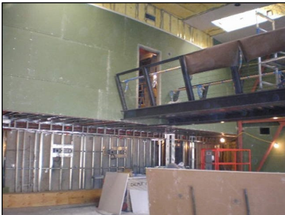
Installing Drywall at the North Side Addition
