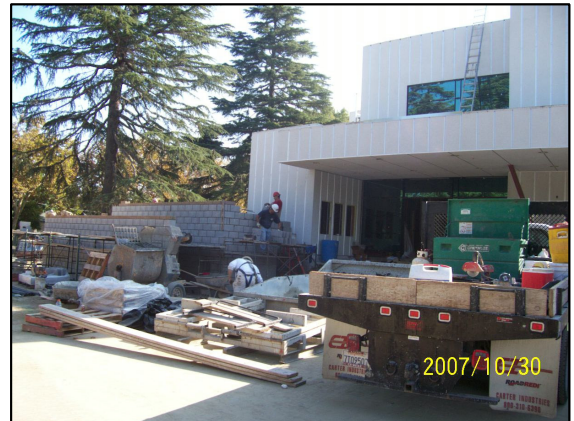
Building CMU Walls at the North Side Addition
