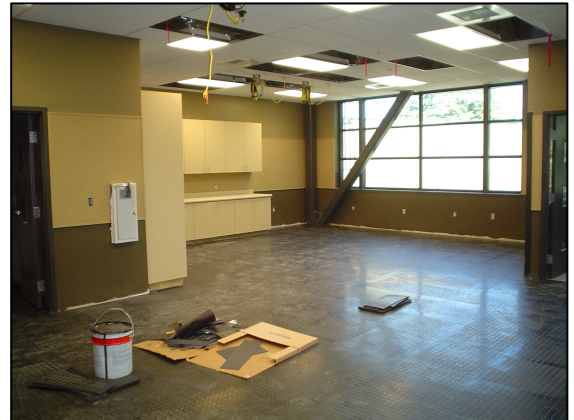
Setting Rubber Tile in the Costume Construction Shop
