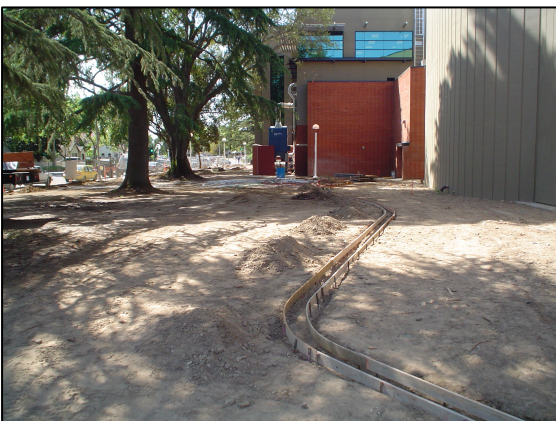
Forming Mow Strips at the North Side Addition
