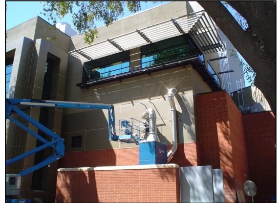
Installing Ductwork at Dust Collector Unit
