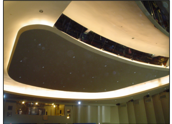
Testing the Dim Cove Lighting System
