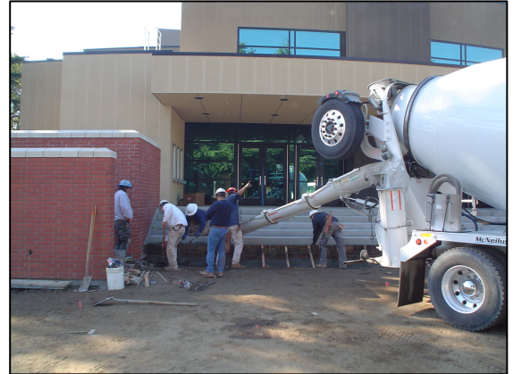
Pouring Exterior Stair at the Front Entry
