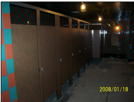
Installing Toilet Partitions in the 2 nd Floor Restrooms
