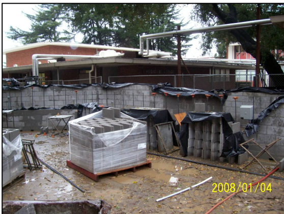
CMU Walls at the West Side Stairs and Ramp
