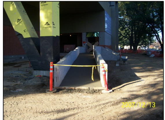
Pouring Ramp at the Loading Dock
