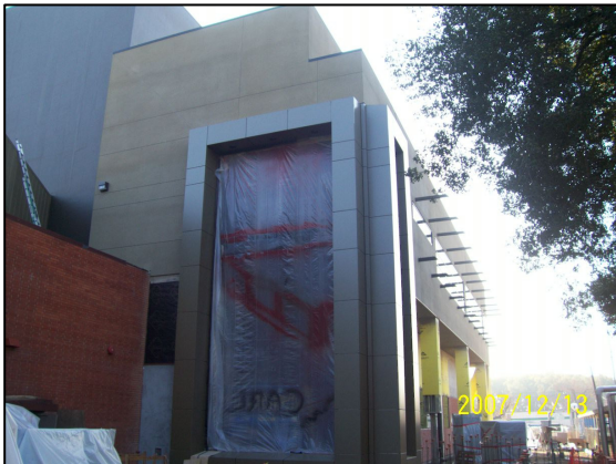
Installing Composite Panels at the South Side Addition
