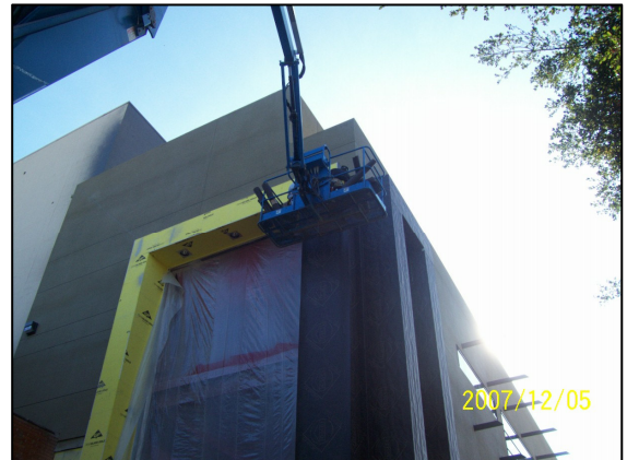
Installing Composite Panels
