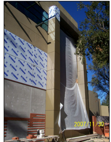
Installing Composite Panels
