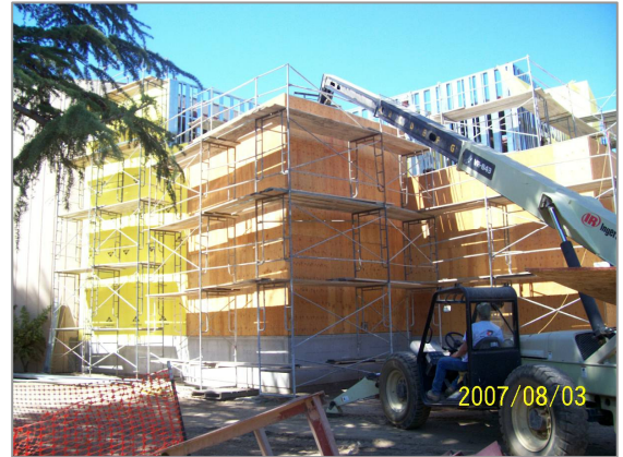
Sheathing Exterior Walls at North Side Addition
