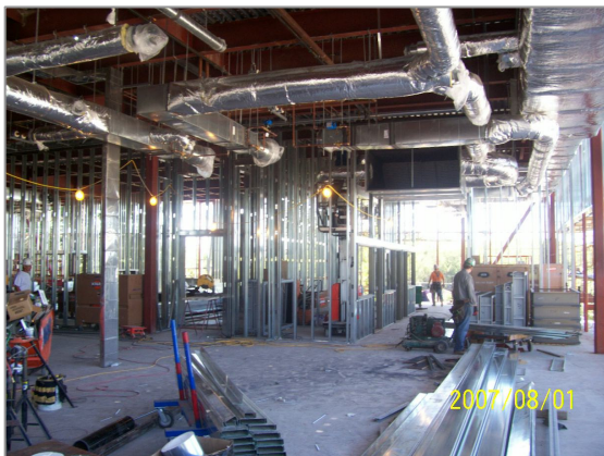
MEP Rough-in at the 2 nd Floor of South Side Addition
