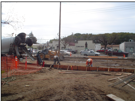
Pouring Curb & Gutter at the New South Side Parking Lot
