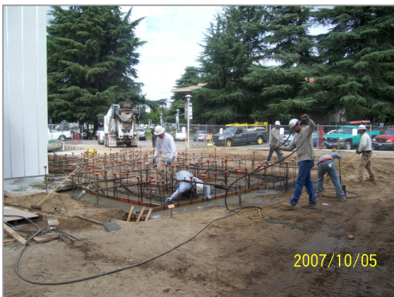
Pouring Exterior Footings at the North Side Addition
