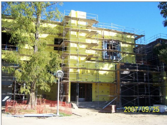
Lathing Exterior Walls at the South Side Addition
