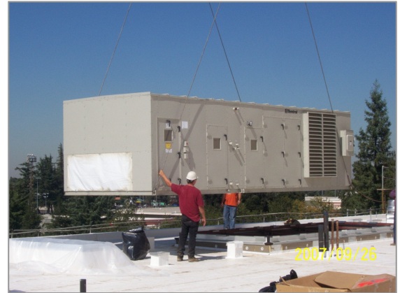
Installing Roof Top HVAC Units at the South Side Addition
