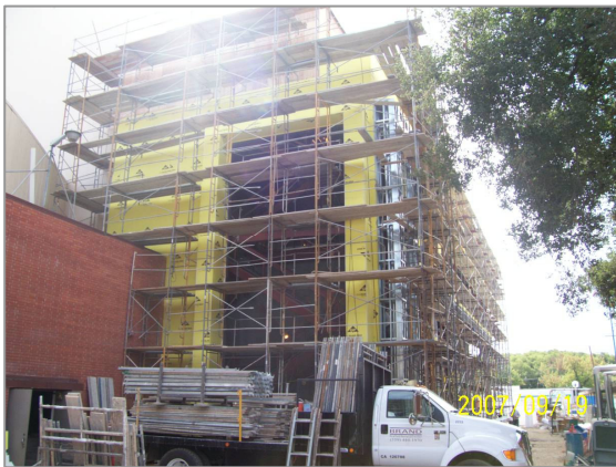
Sheathing Exterior Walls at the South Side Addition
