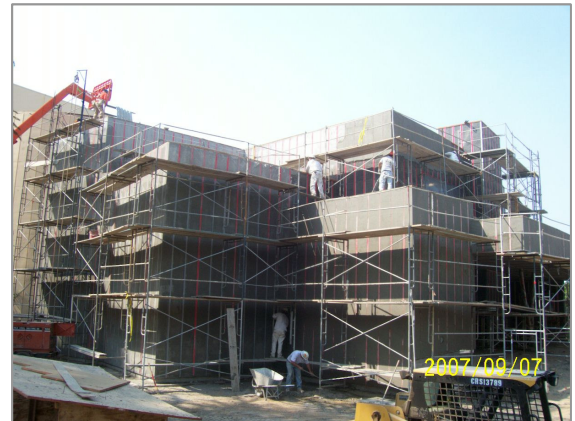
Plastering North Side Addition Exterior Walls
