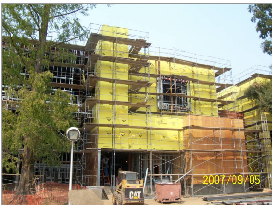
Sheathing South Side Addition Exterior Walls
