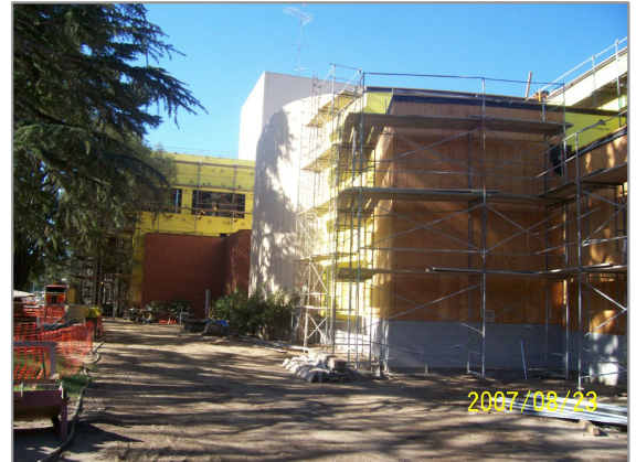
Sheathing East Side Exterior Walls
