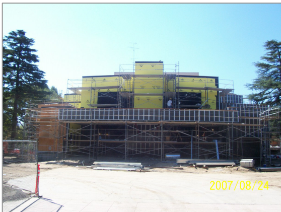
Installing Trim & Lath at the North Side Addition
