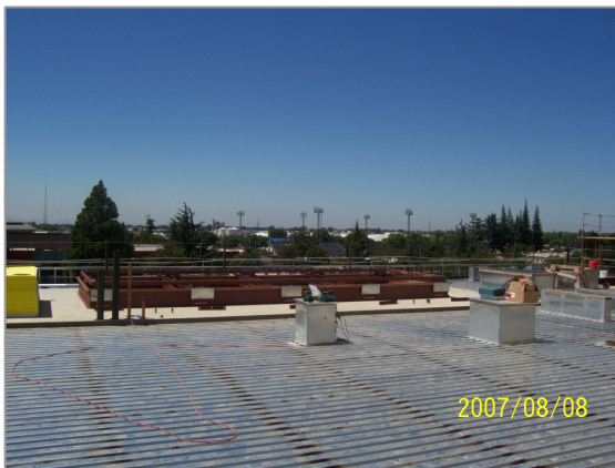
Installing Roof Top HVAC Equipment
