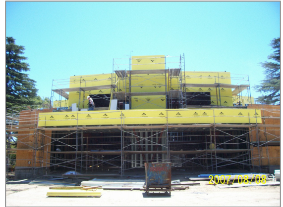
Sheathing Exterior Walls at North Side Addition
