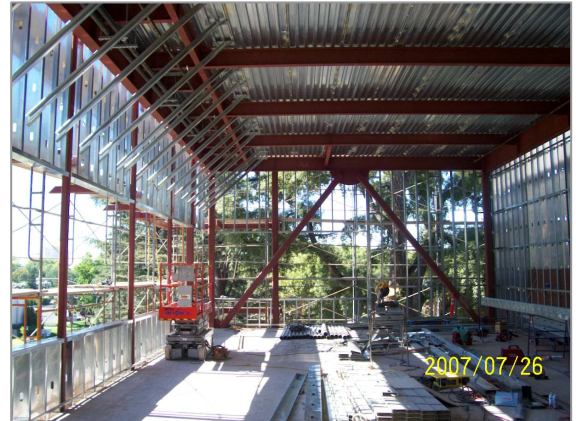
Framing Rehearsal/Multipurpose at 2 nd Floor of South Side Addition
