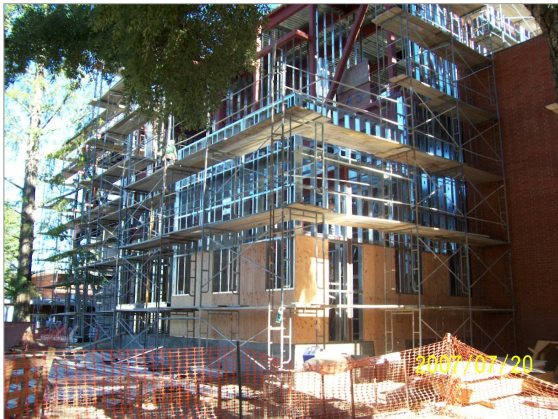
Sheathing Exterior Walls at South Side Addition
