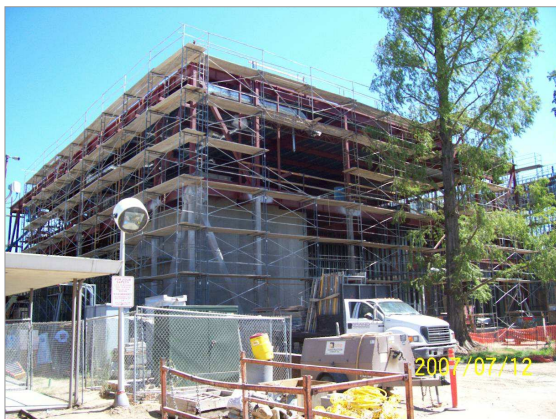
Erecting Scaffold at South Side Addition
