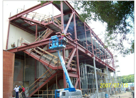
Welding Storefront Steel Support
