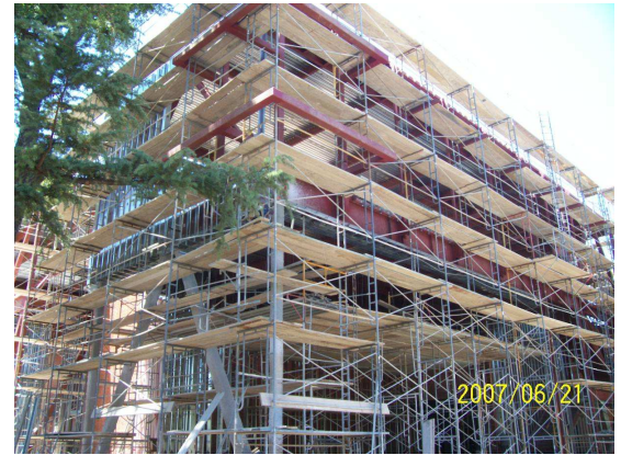
Framing Perimeter Walls at South Side Addition
