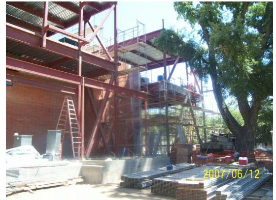
Scaffolding at South Side Addition
