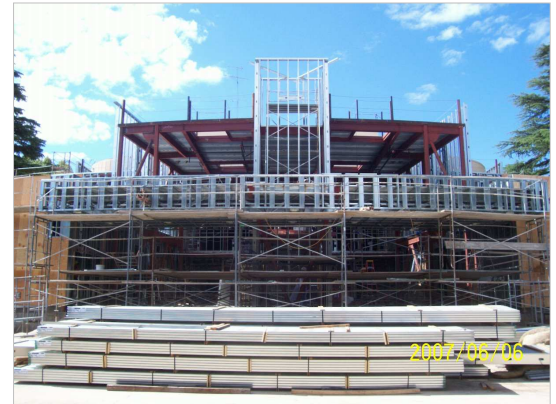
Lath for Installation at North Side Addition
