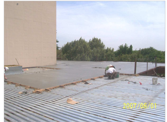
South Side Addition Concrete Roof Pads
