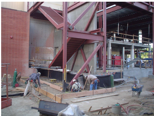
West Side Stairs and Footing Form Installation
