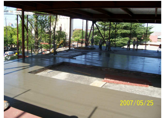
Placing South Side Addition 2 nd Floor Concrete
