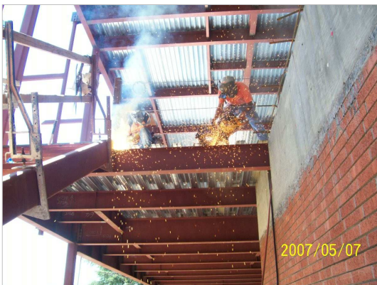
Cutting Metal Deck at South Side Addition
