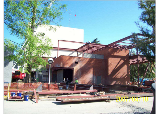
South Side Addition Structural Steel
