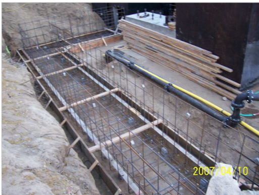
Formwork for West Side Tunnel Floors
