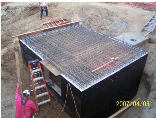
Top Reinforcement for West Side Vault
