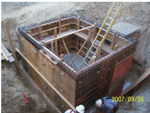
Wall Forms for East Side Vault
