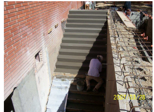
Finishing East Side Stairs to Basement
